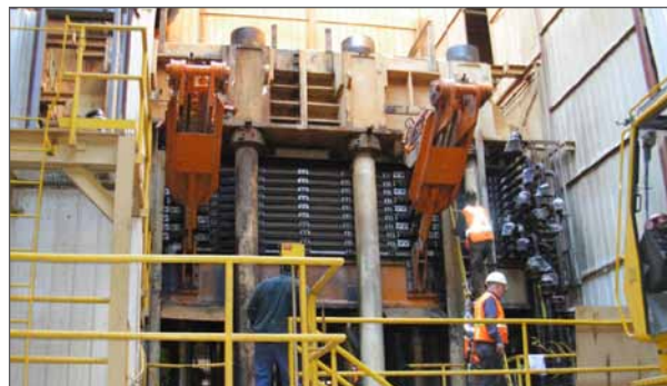
Above is an example of a customer field testing application in the construction industry. The Rexnord Innovation Center was enlisted to explore column failures in a forest products processing plant.
