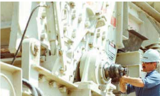
Field installation of condition monitoring devices on portable crushing plant
