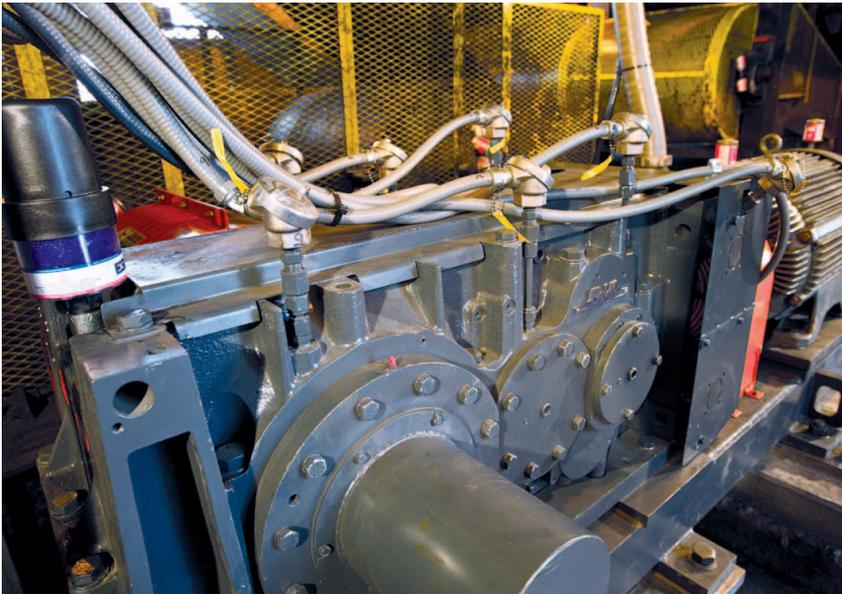
Figure 2. The 324 hp. Falk V-Class with split shaft fan and condition monitoring package.
