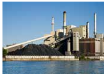
Energy processing equipment
