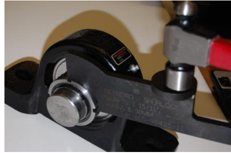
Figure 4: Tightening Locknut using Impact Wrench
