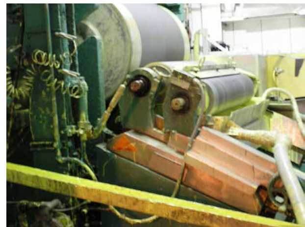
Applicator rollers in operation
