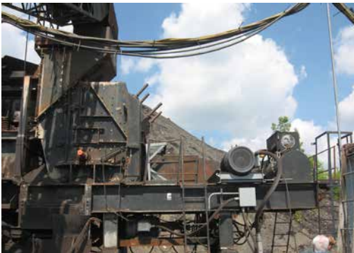
Large crusher used for asphalt recycling at Eureka Stone's Rushland, PA plant was converted from diesel to electric drive, using Rexnord SHURLOK Bearings and Omega Coupling on the jackshaft.
