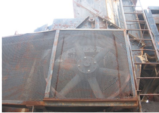
View from opposite side shows large multiple V-groove pulley that drives the crusher (inside guard).
