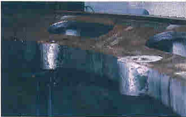
Completed Weld Repair
